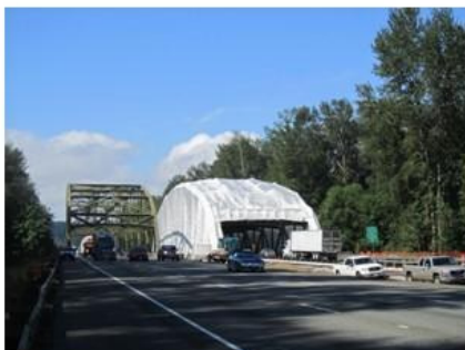
I-5 Nisqually River Bridge near Olympia Painted in 2014
