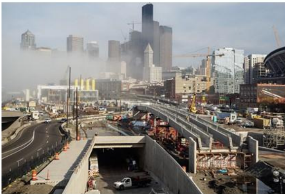
SR99 – Entrance to new Alaskan Way Tunnel
