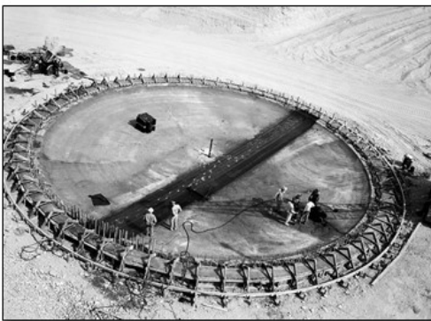
Tank foundation under construction.
