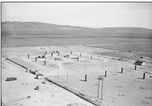
Tanks are underground to shield radiation.
